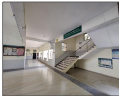
Staircase with Railings
